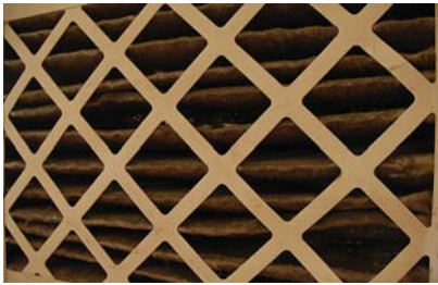
Used air filter. Source: MosArt Architecture.
