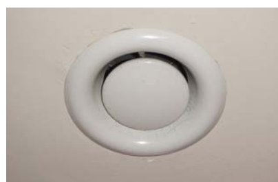
Ceiling air supply vent. Source: MosArt Architecture.
