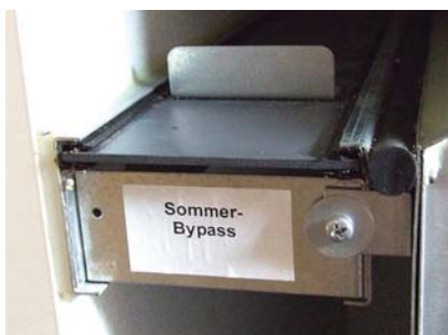
The sommer-bypass can be used for cooling in the summer if needed. Source: MosArt Architecture.
